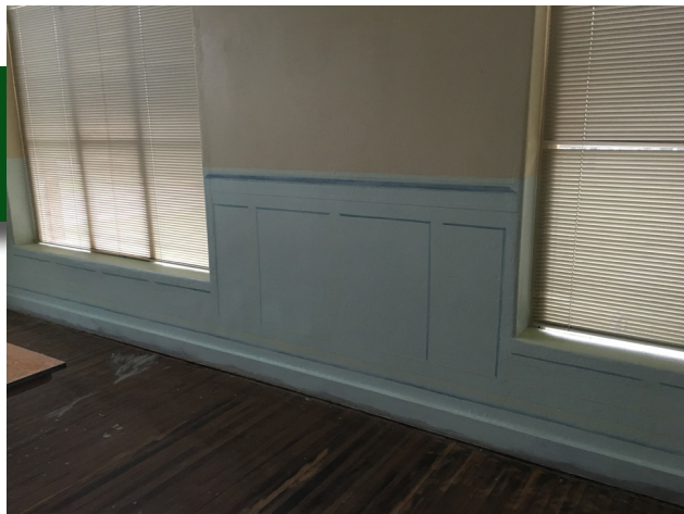
Walls after plaster repair and paint
